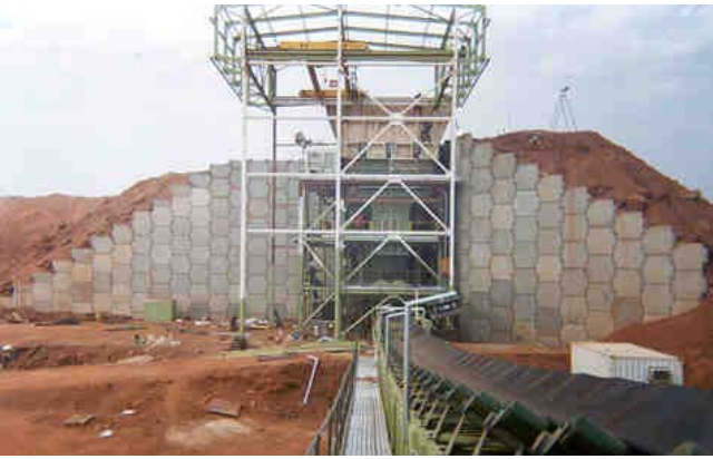
Figure 4. Precast concrete cladding – Siguiri Mine, Guinea
