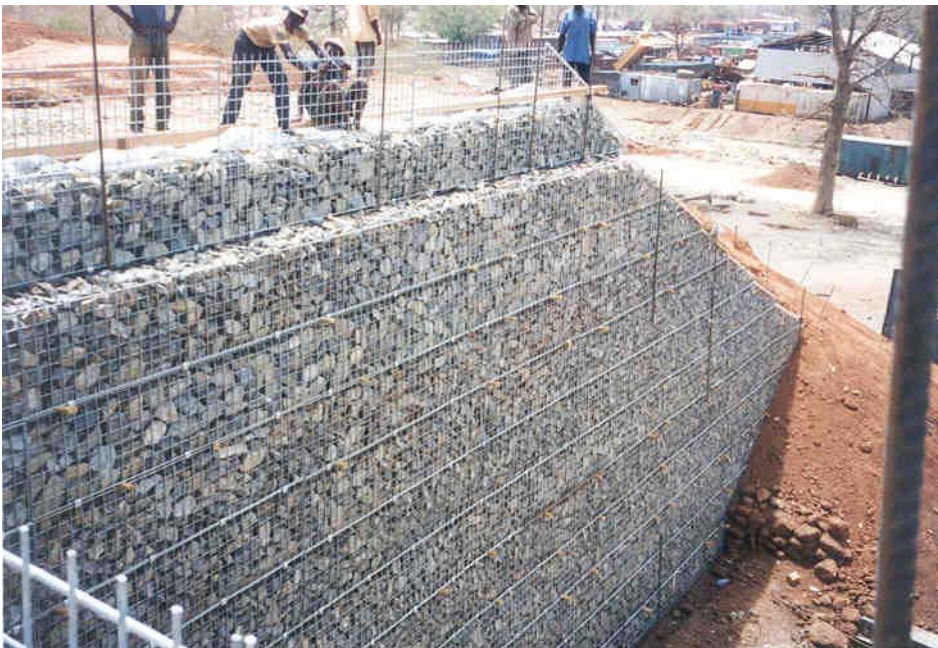
Figure 2b. Weldmesh cladding backed with rock – Sadiola Gold Mine, Mali
