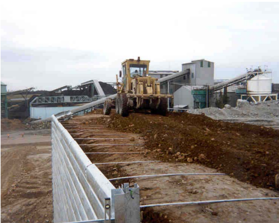
Figure 3b. An example of a steel cladding wall as used at Miba Mine above .
