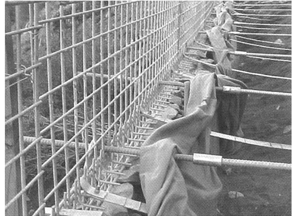
Figure 4. Detail of the nail extension.
