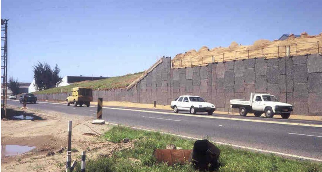
Figure 9. An abutment prior to construction of distribution beams
